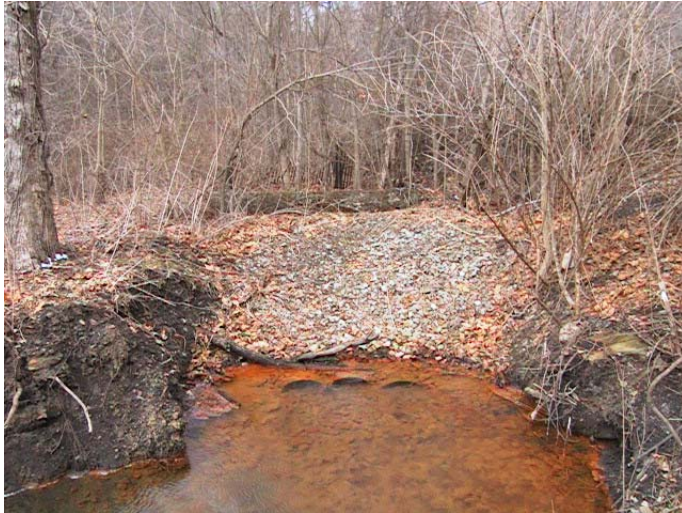
Figure 1. The Marchand Mine discharge. Flow is through three pipes that extend through aggregate placed in the entry.
