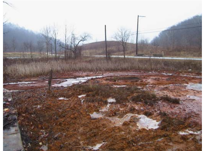
Figure 2. The sludge-filled channel before processing activities.
