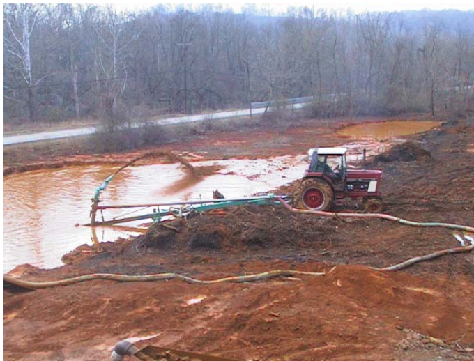
Figure 4. Sludge removal with a tractor pump.
