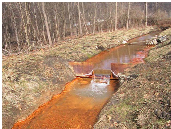
Figure 3. The discharge was relocated to a new channel during processing. A weir was installed in the channel.
