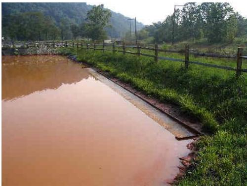
In autumn 2006 the world's first passive mine water treatment system designed to produce a clean saleable iron oxide product became operational. The system is located in Lowber PA (Westmoreland County) and treats a 1,400 – 2,400 gpm discharge of iron-polluted water from the abandoned Marchand coal mine.
