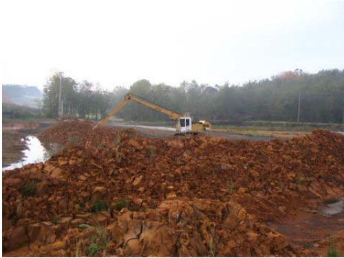
installation of a treatment system, iron sludge from an existing pond was pumped into sludge disposal basins. In August, IOR mobilized in its newly purchased Priestman excavator and began to dewater the sludge through stacking and windrowing. In July truckloads of material began to leave the site for delivery to the Clarion processing plant or to Hoover Color Corporation. As soon as
